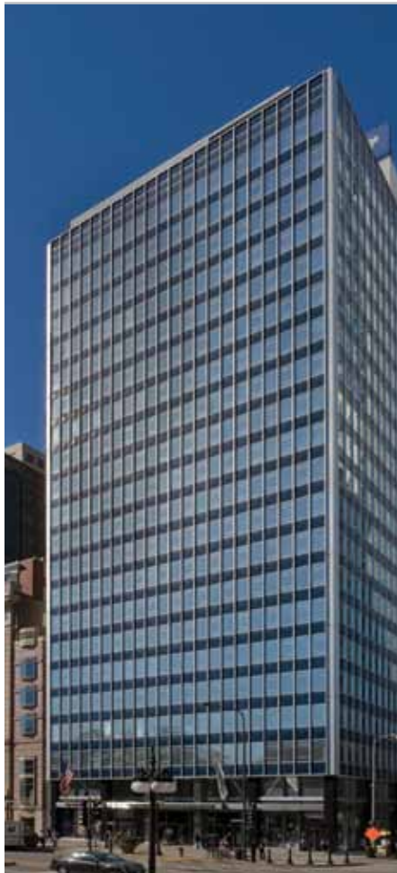
200 South Michigan Avenue, Chicago, IL
