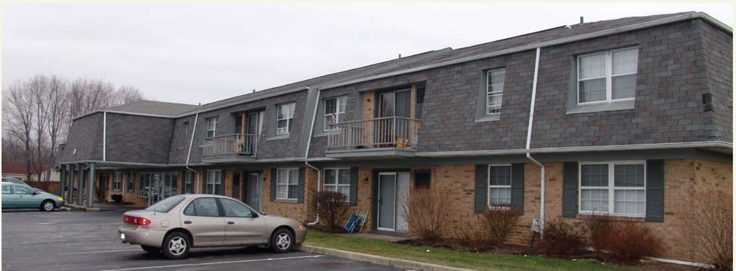
Dogwood Gardens, East Norriton, PA - Before Renovations
